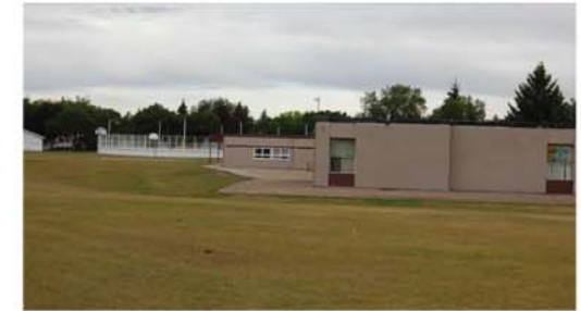
J. Low lying area at southwest corner of school.
